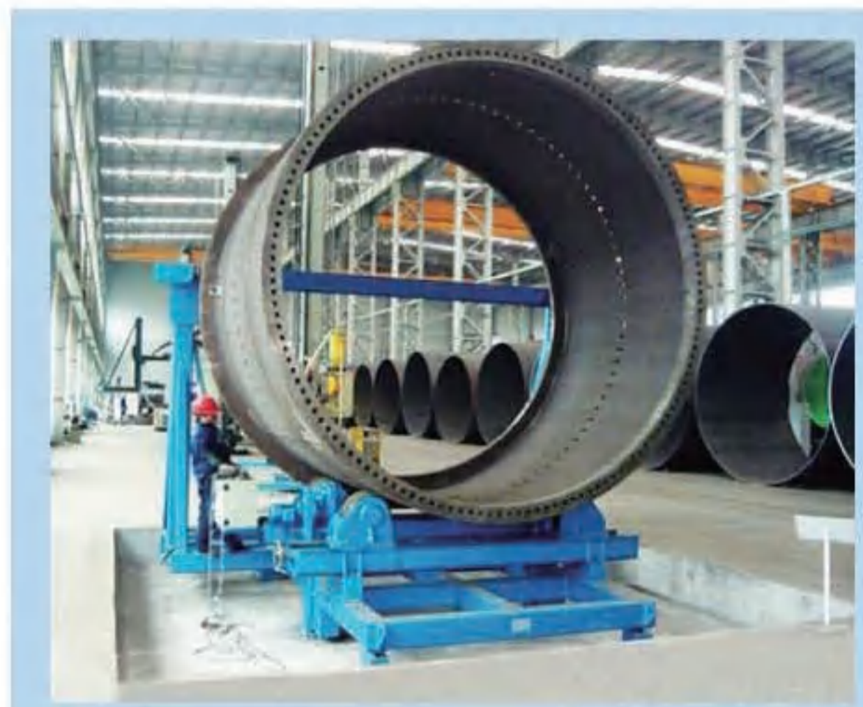
塔筒外环焊接 Outer circumferential welding
