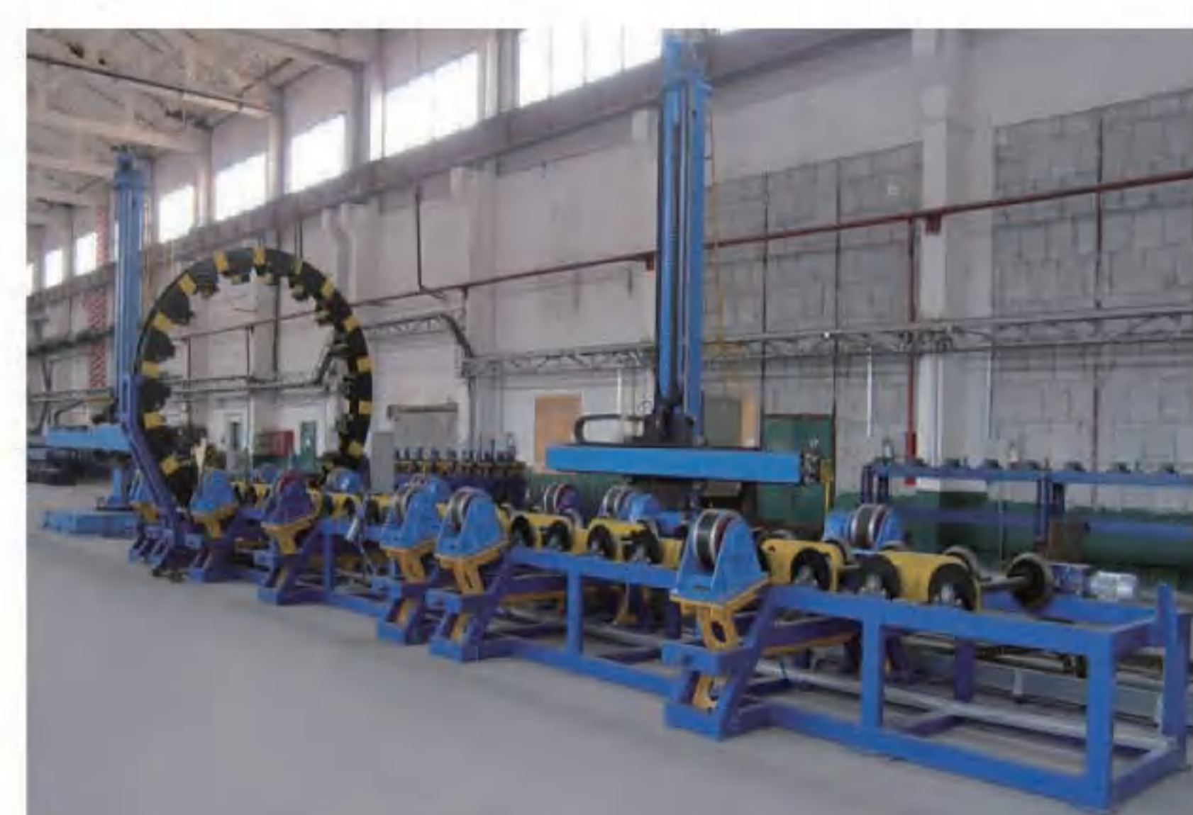
筒体焊接流水线 (定制) Simplified welding assembly line (custom)
